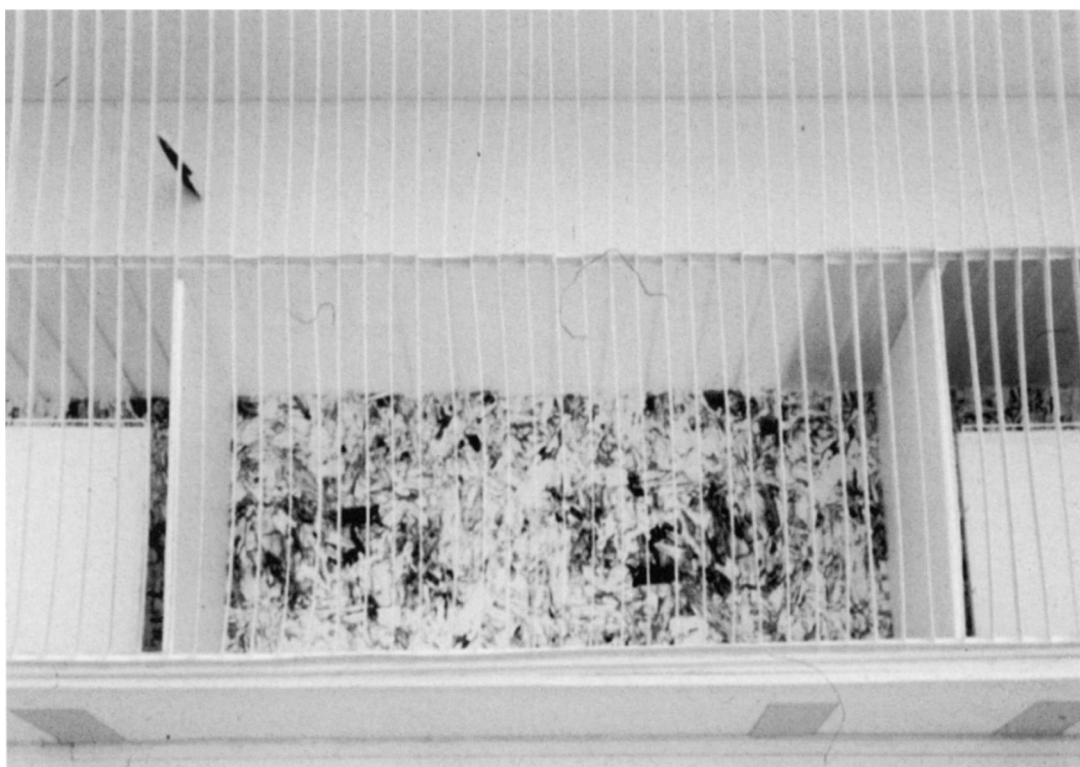
View of interior from above
